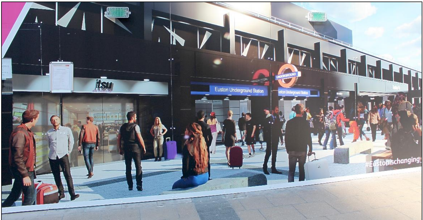
Above: A new entrance for the Underground is under construction at Euston, at the front of the main line station, this being on a hoarding protecting the incomplete new entrance behind.
